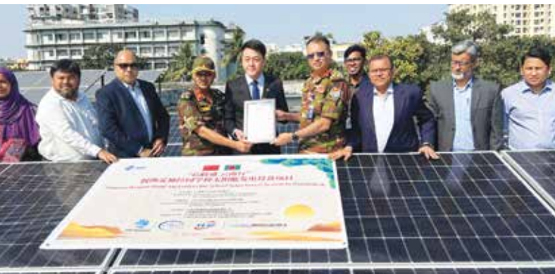
Figure: Brig. Gen. Kazi Shameem Farhad and Brig. Gen. Muhammed Zaber Hossain, Principals of Dhaka Residential Model College inaugurated the 23.2 kWh rooftop solar project
